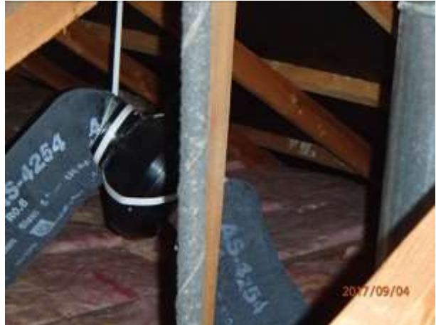
Bathroom extract duct to outside. Heat transfer has a bend that is probably restricting flow
