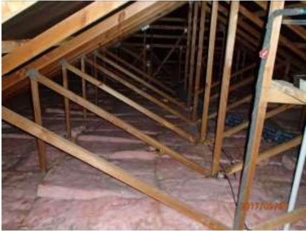
The batts and header tank are all tidily installed
