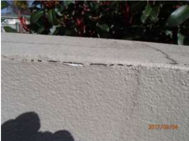
Cracks in the wall are letting a lot of water in, would have been better if only one side was plastered because the timbers could have a chance to dry out.
