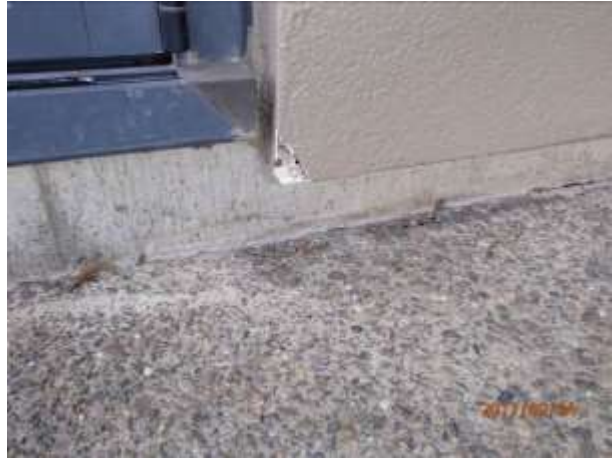
Minor damage to some corners just needs to be repaired before repainting.
