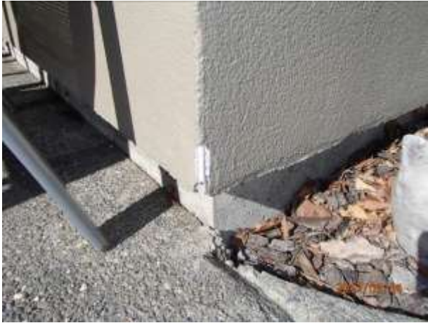
Minor damage to some corners just needs to be repaired before repainting.
