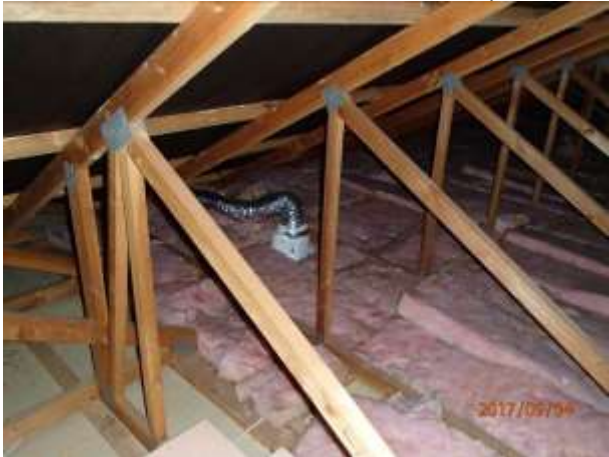
Bathroom extract duct to outside. Heat transfer has a bend that is probably restricting flow
