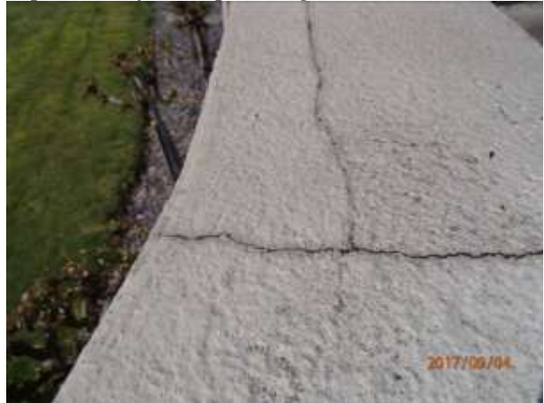
Cracks in the wall are letting a lot of water in, would have been better if only one side was plastered because the timbers could have a chance to dry out.
